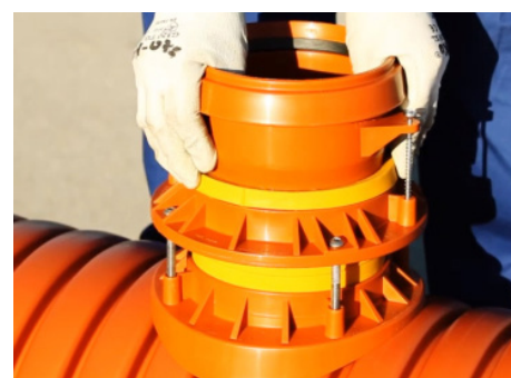
9 Serraggio viti autofilettanti 9 Tightning of self-tapping screws
