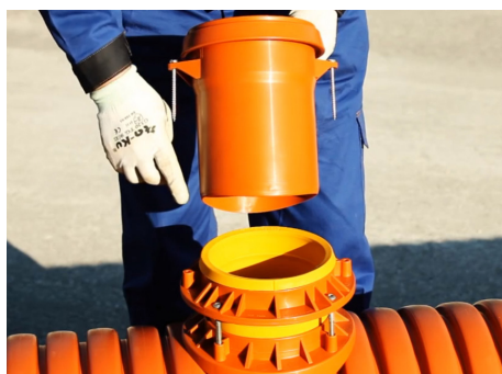
8 Inserimento codolo 8 Application of socket
