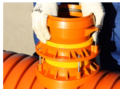
9 Serraggio viti autofilettanti 9 Tightning of self-tapping screws
